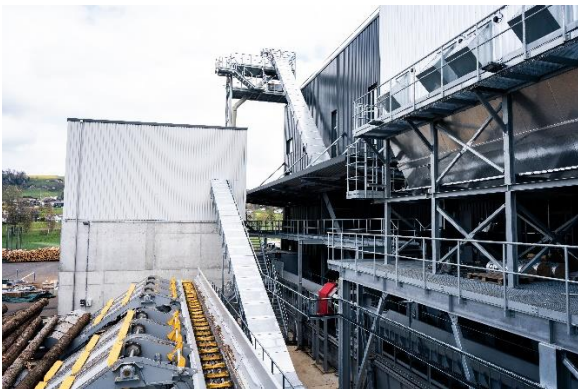
Photo 6: The waste bark collected in the box is also transported to the pellet facility.
